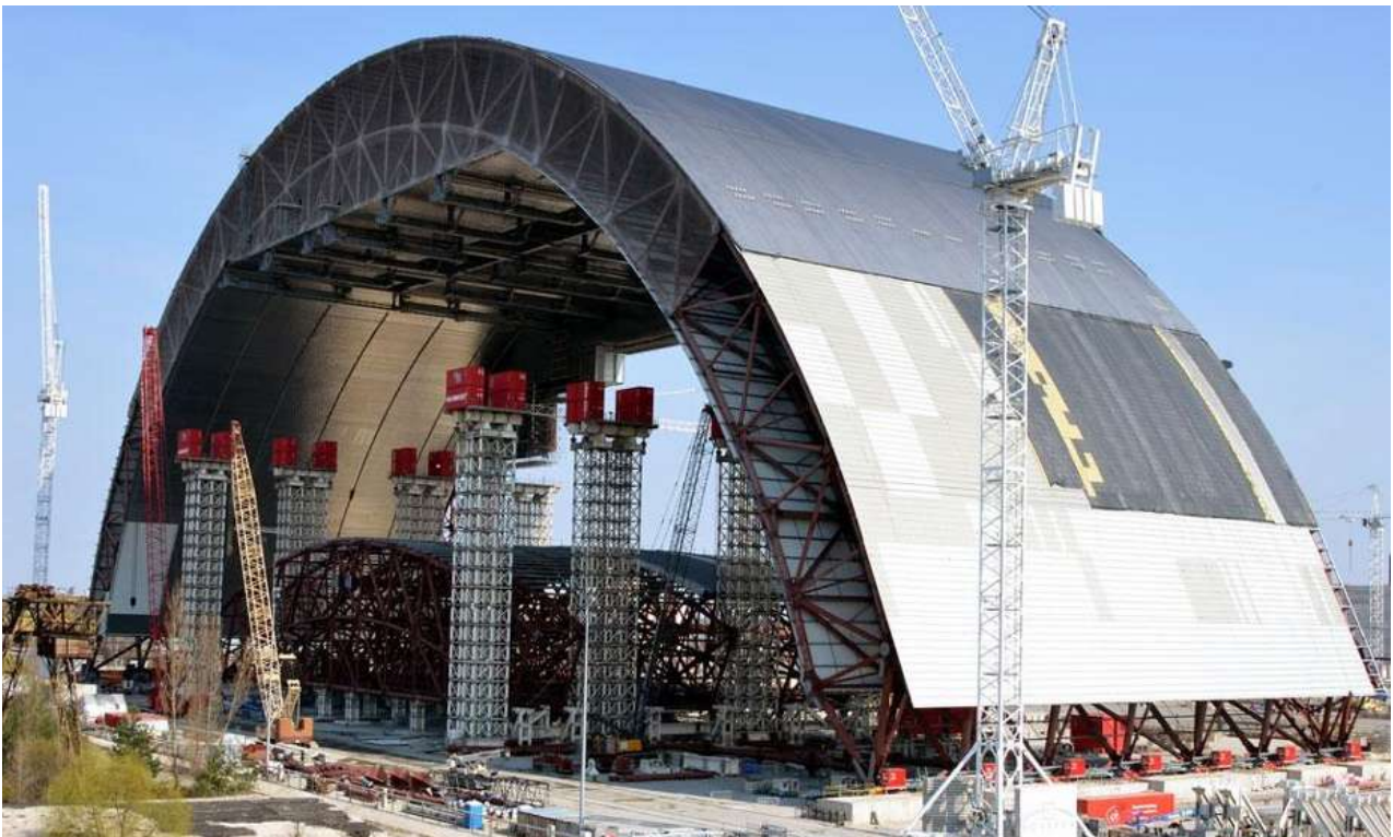
NSC structural members and inner/outer shells during construction - Credit EBRD
